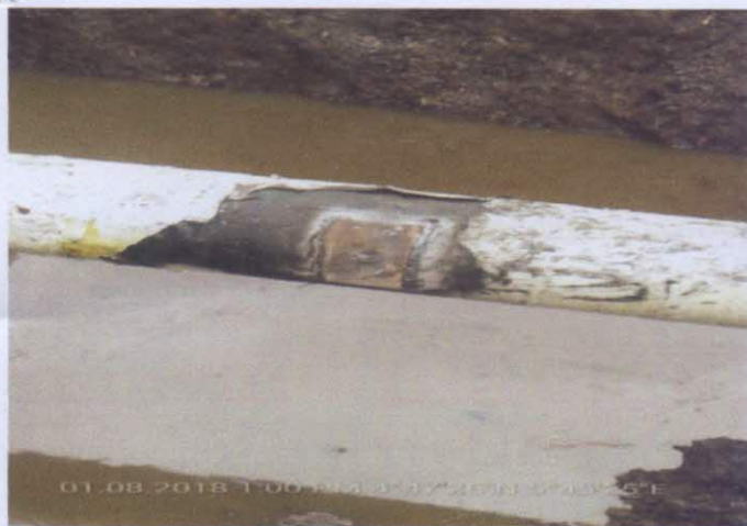
Figure 3: welded section on the Pipeline.
